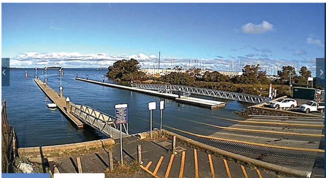
Hastings Boat ramp, upgraded.
